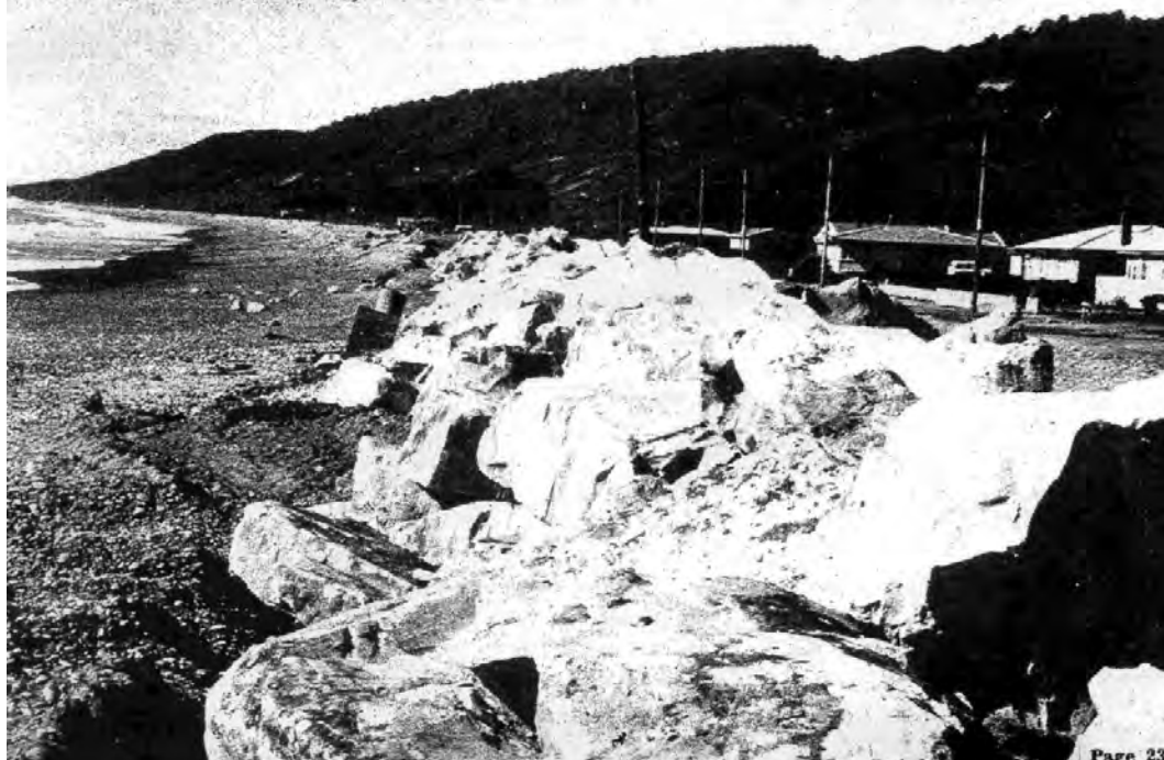
Down goes several tons of rock on to the de protection works. Below: Some idea of the the undertaking is given by this shot of the
