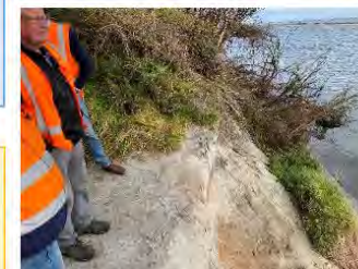
Okuru River Mouth erosion adjacent to road
