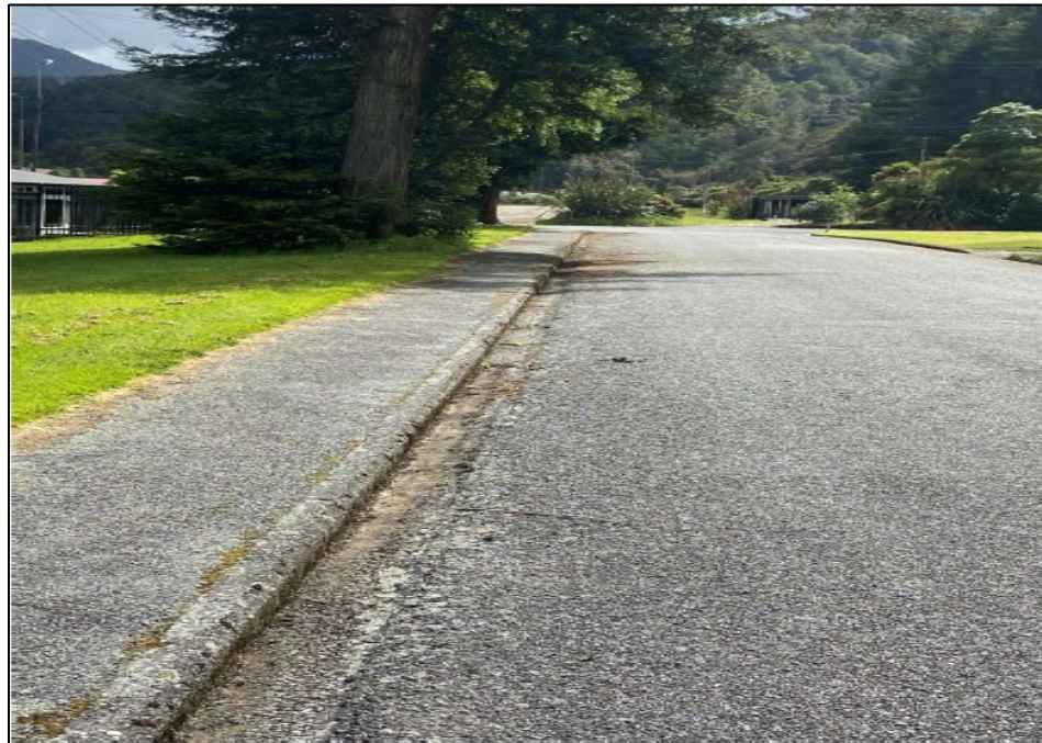
Fig 2: Kerb and Channel cleaning works
