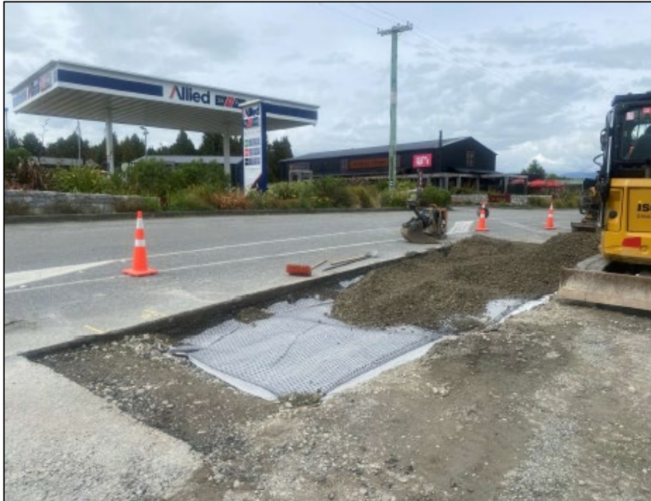
Fig 1: Pavement repair works at Arnold Valley Road at Moana
