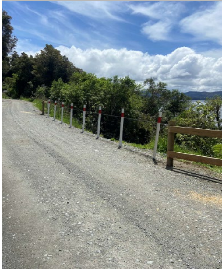
Fig 3: Temporary Safety Improvement works on Kumara – Inchbonnie Road
