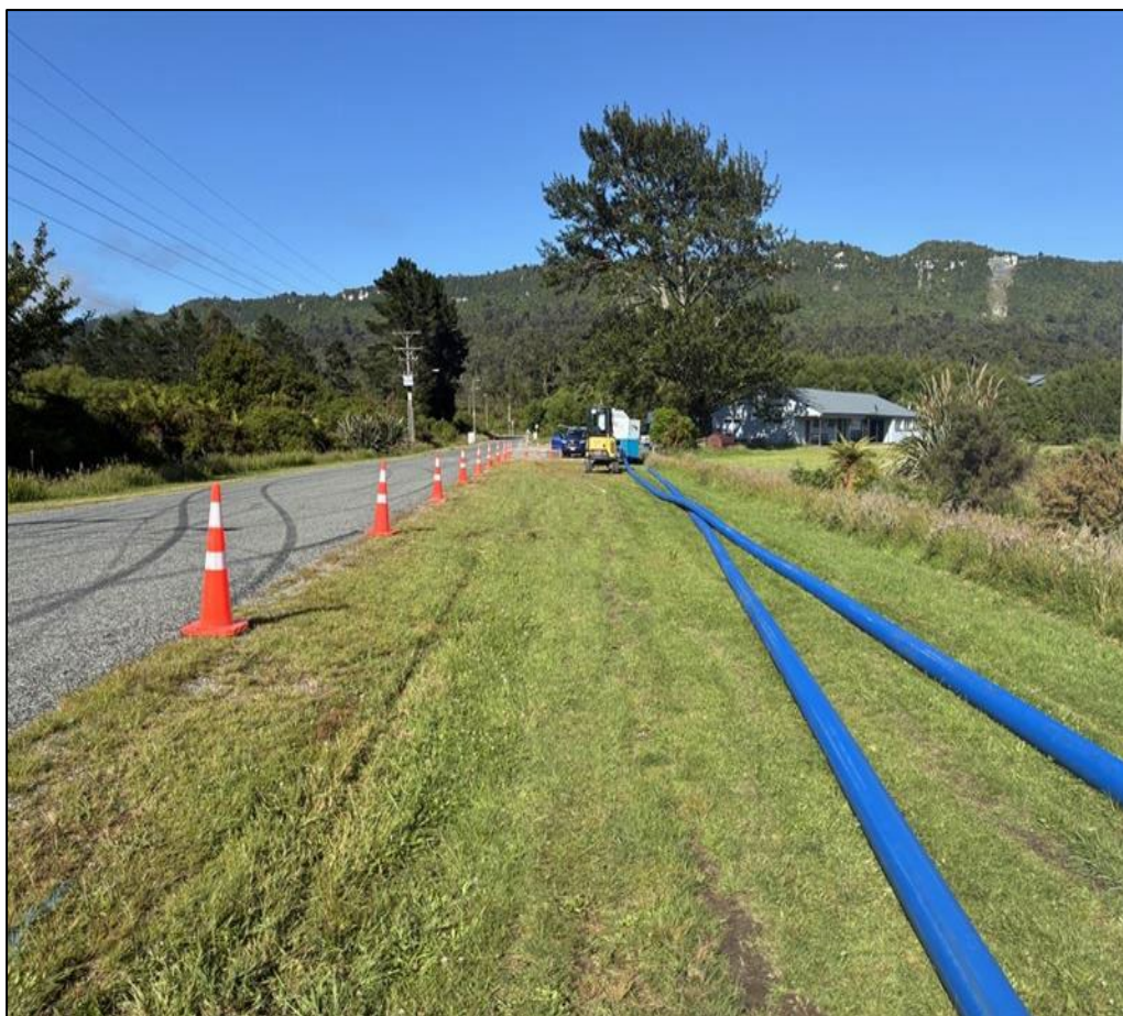
Fig 5: Water Main Pipe Laying at Somerled Ave
