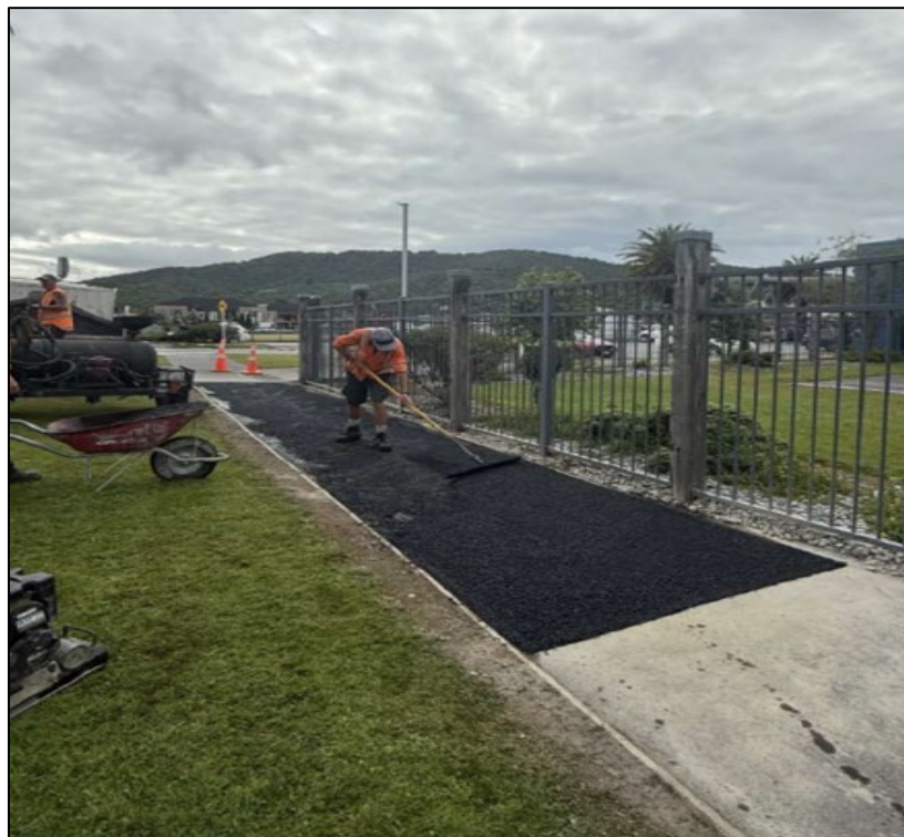
Fig 3: Footpath Renewal on High Street
