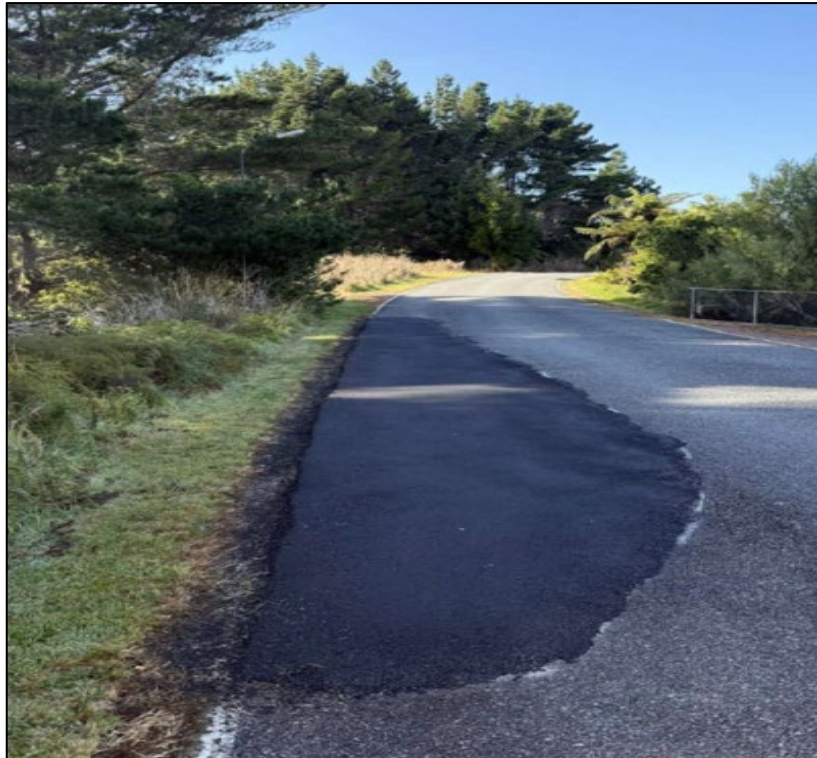
Fig 2: Pavement repair works at Tasman View Road
