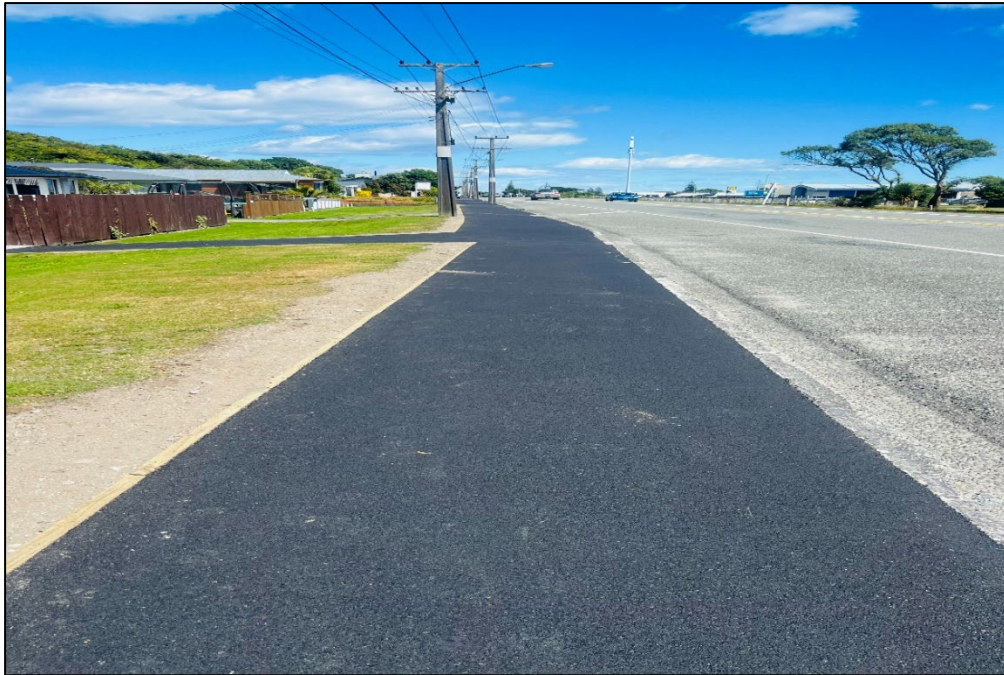
Fig 8: Footpath Renewal works on High Street
