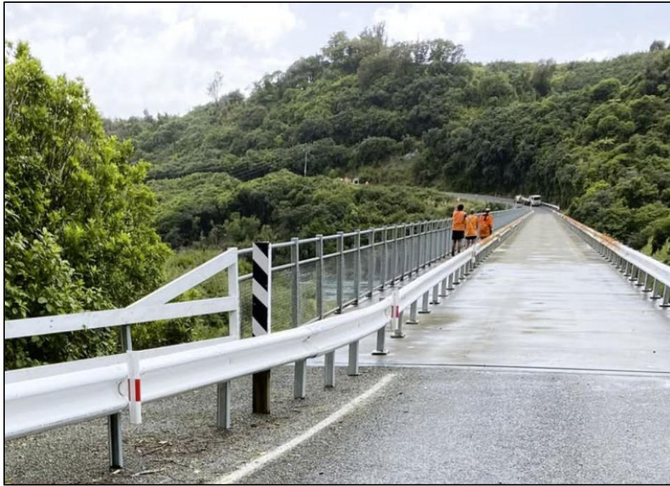
Fig 6: Painting works completed on William – Stewart bridge
