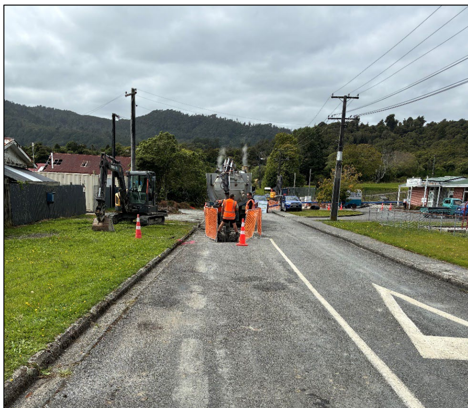
Fig 7: Runanga Wastewater Renewal works on Carroll Street. A road closure was in place at the time of this photo.
