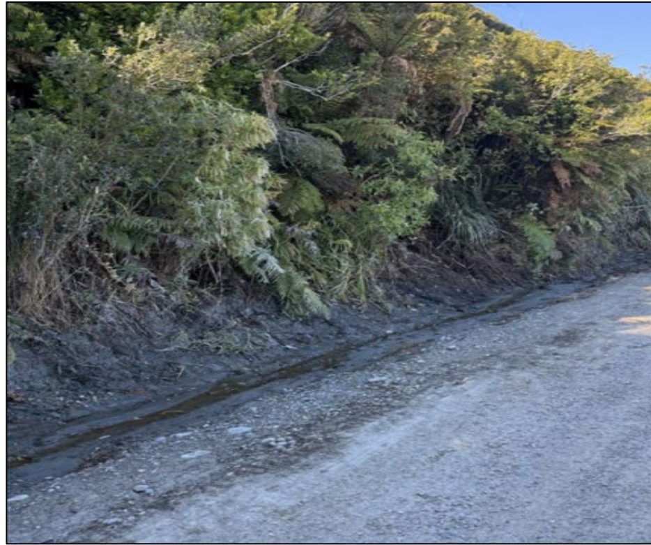
Fig 4: Drainage cleaning works on Neilson Road
