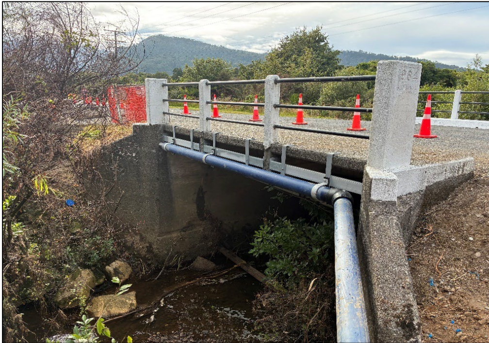
Fig 5: Water Main Pipe Laying (Bridge Crossing) at Somerled Ave
