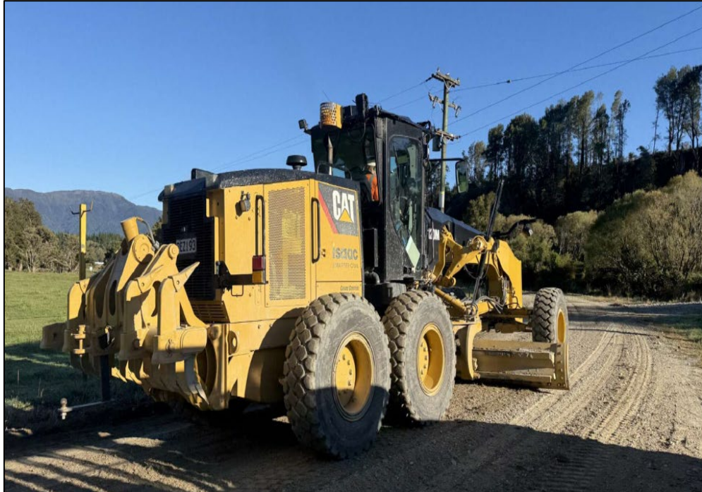
Fig 5: Unsealed Pavement Maintenance works on Red Jacks Road
