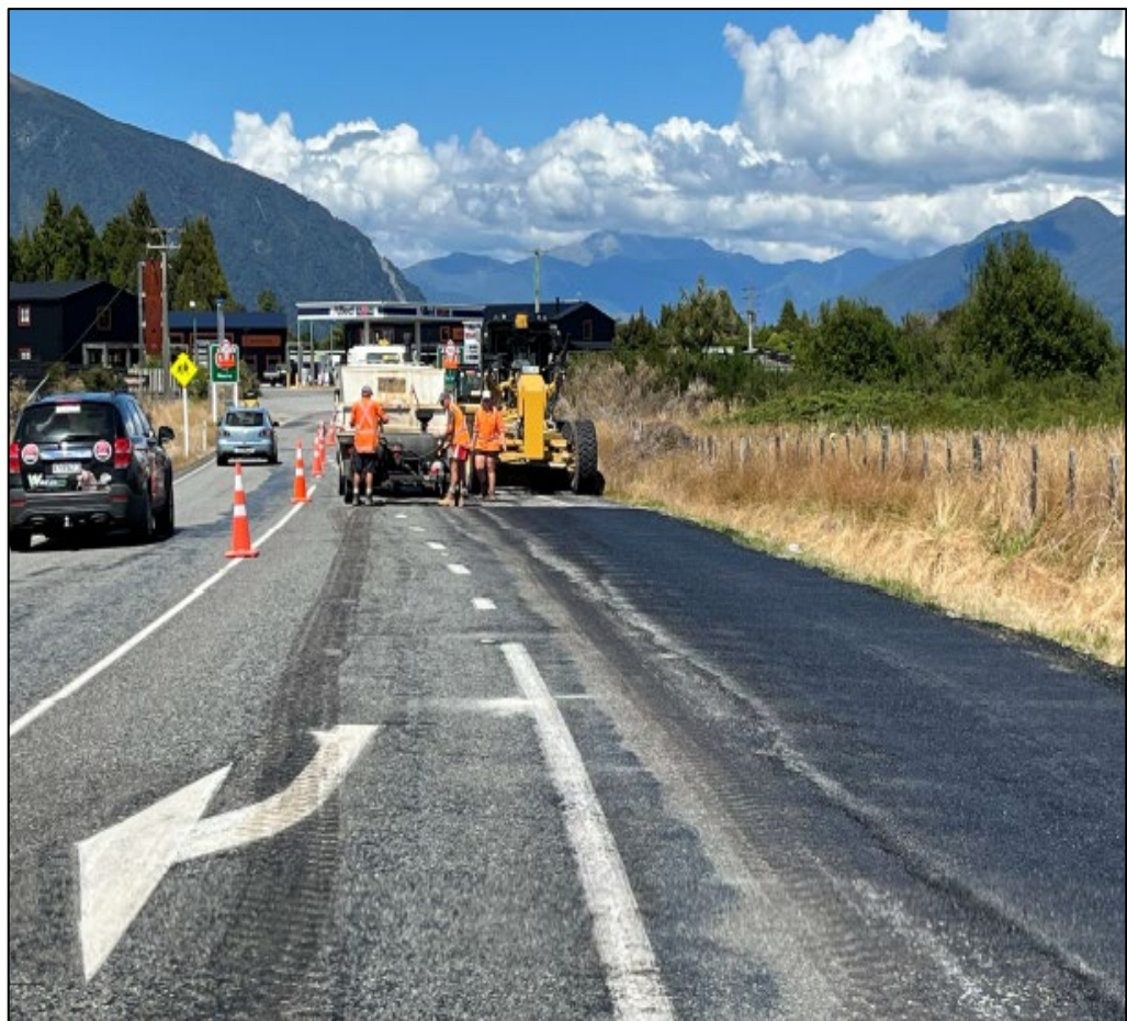
Fig 1: Surface repairs in Moana
