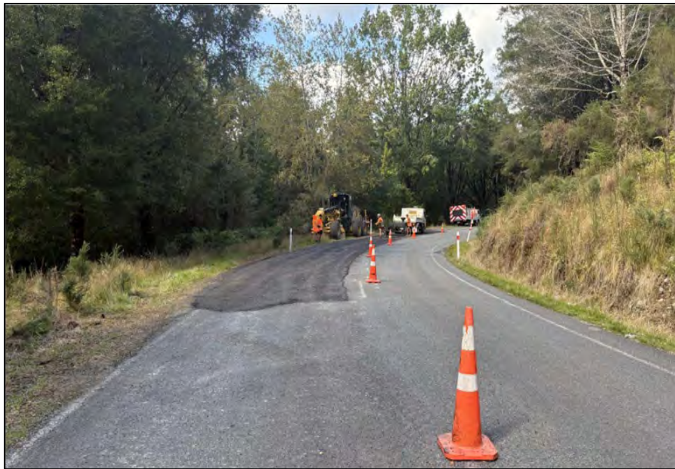
Fig 2: Pavement repair works on Nelson Creek Road
