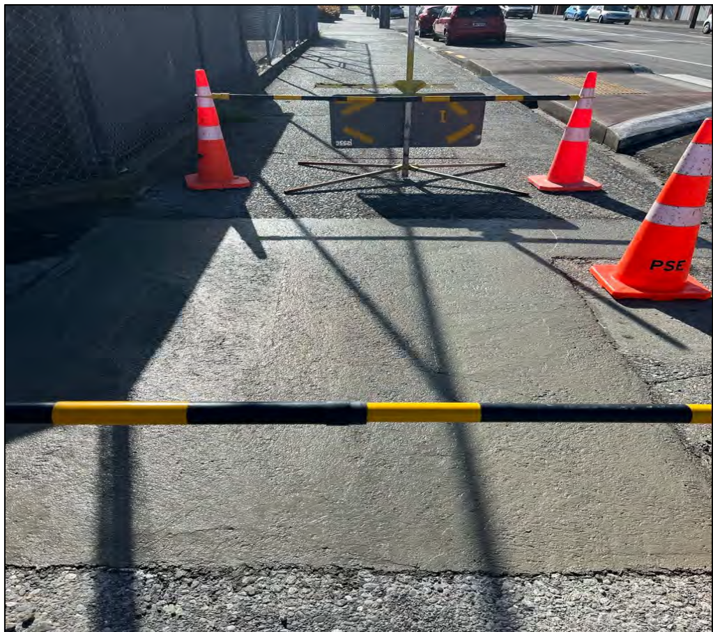
Fig 3: Footpath Renewal on Shakespeare Street
