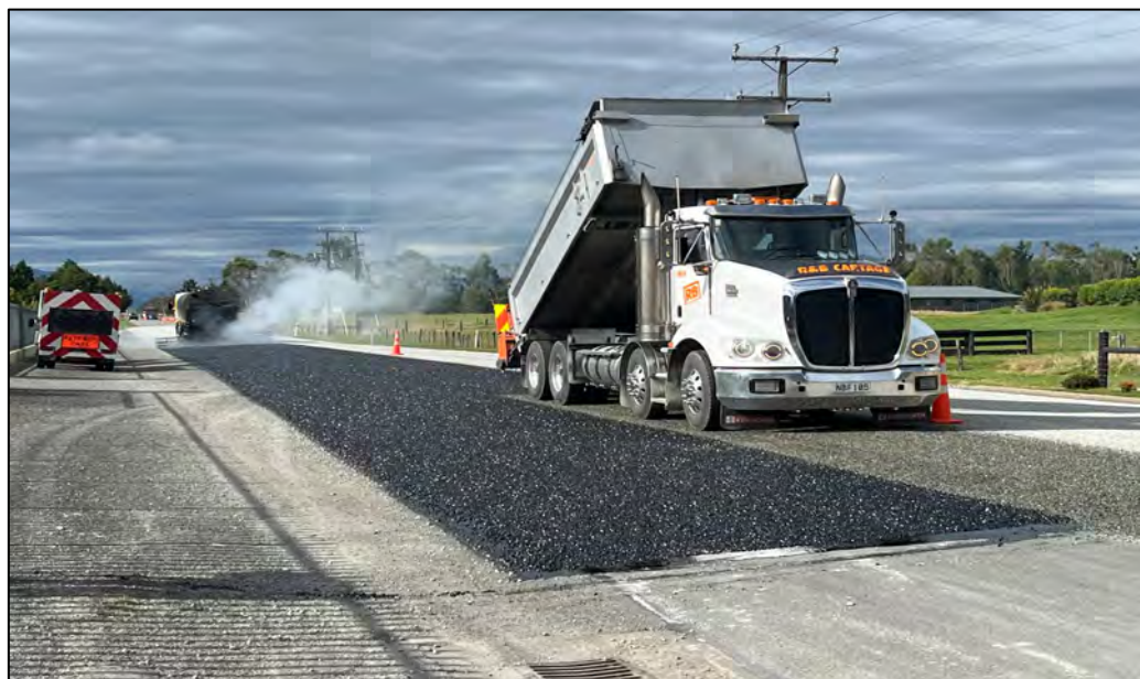
Fig 5: Sealing works on Taylorville Road
