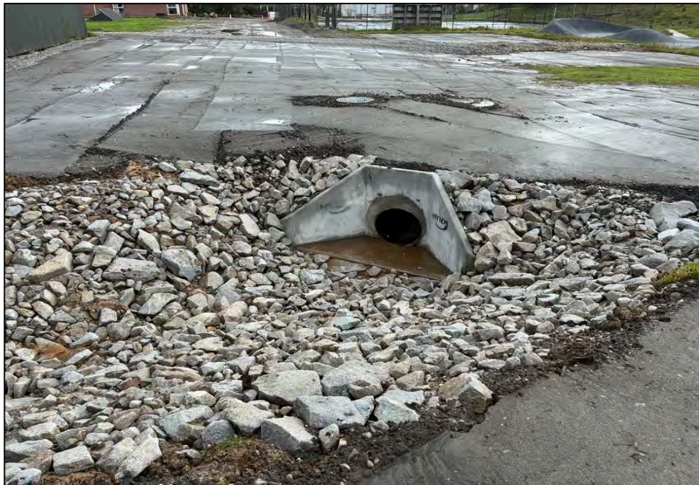
Fig 11: Runanga Stormwater Improvement works on Kotare Domain area.
