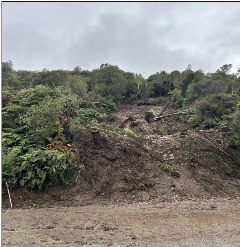
Fig 6: Slip on Taylorville Road
