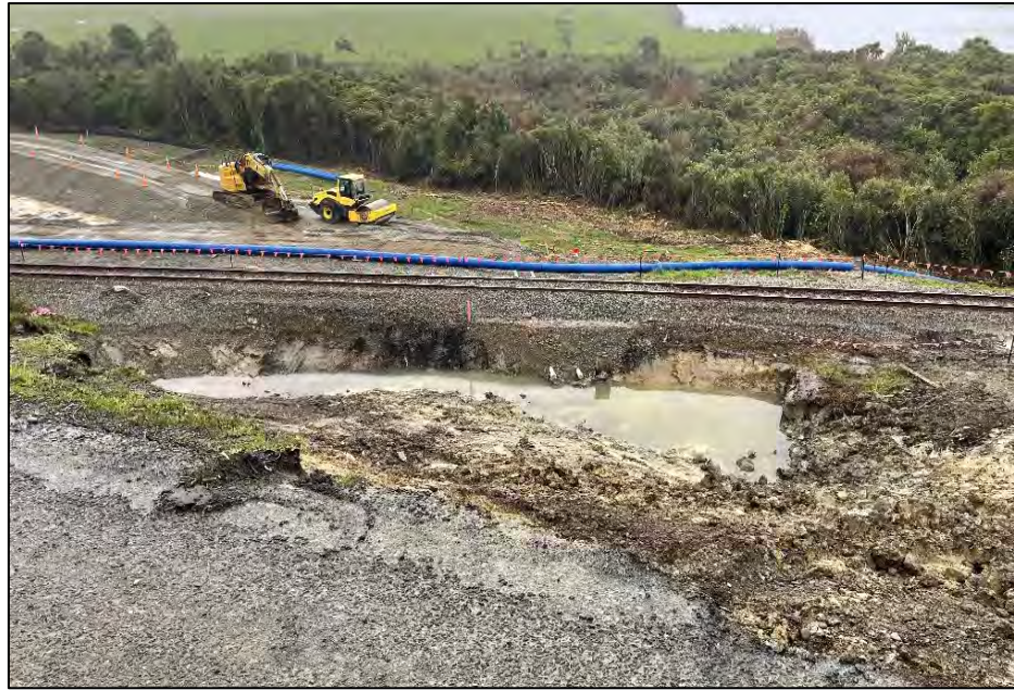
Fig 7: Site photo near SHWY temporary bypass road.
