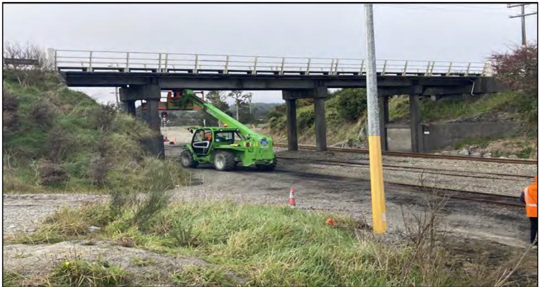
Fig 2: Works on Stillwater Railway Overbridge
