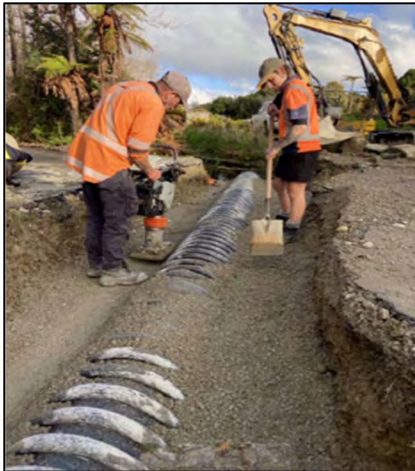
Fig 1: Culvert Replacemet works on Salt Water Creek Road
