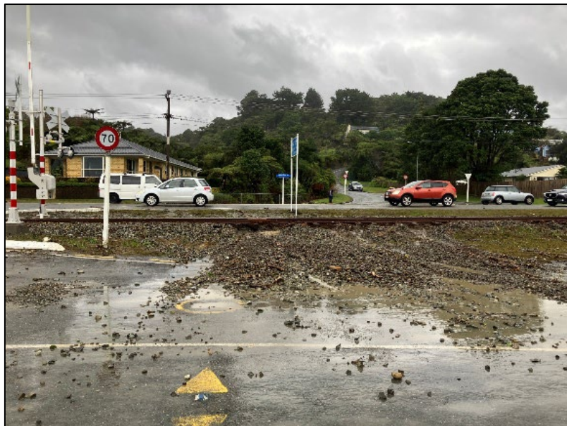
Fig 8b: Rail damage adjacent to the Tasman street/SH6 intersection
