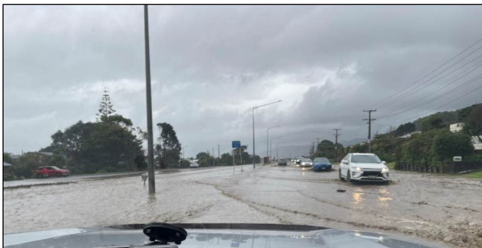
Fig 5: State Highway 6 - Rail line adjacent to Rata Street, Karoro
