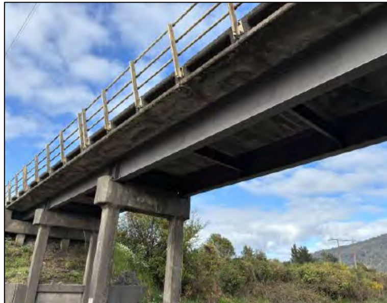
Fig 2: Works on Stillwater Rail Overbridge
