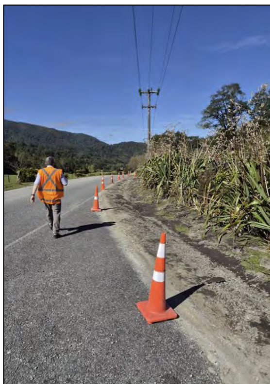
Fig 1: Drainage Renewal Works on Roa Road
