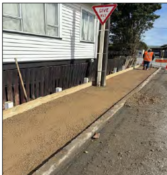
Fig 3: Footpath Extension works on Raleigh Street
