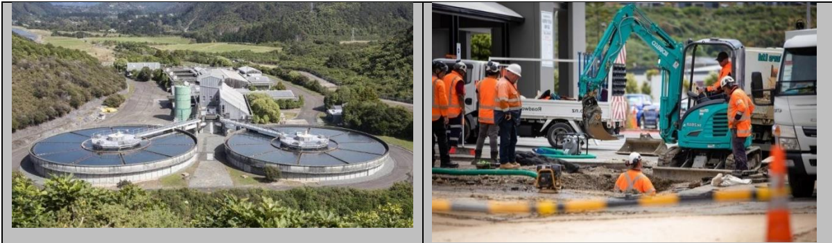
Fig. A3-1 (Left): A Wellington Water fluoridation plant was shut down after an over-dosing incident. Fig. A3-2 (Right): Another challenge for Wellington Water: ageing pipes and associated infrastructure for water, wastewater, and stormwater.
