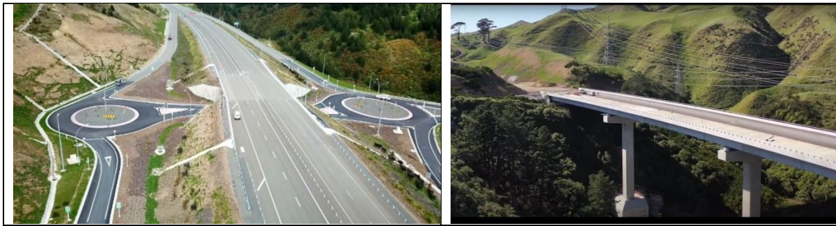
Fig. A3-3. Transmission Gully motorway north of Wellington
