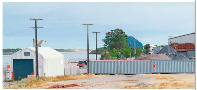
Heavy mineral sand stockpiled on Westport's wharf blew through town in yesterday's strong winds. Photo: Ellen Curnow
