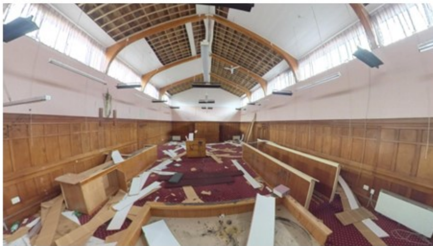
Figure 4 Courtroom timber interior
