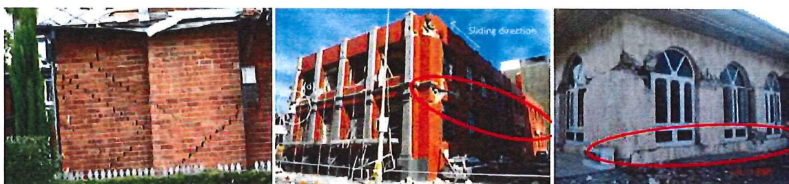
Figure 14. In-Plane Failures of URM Wall (NZSEE Guidelines)
