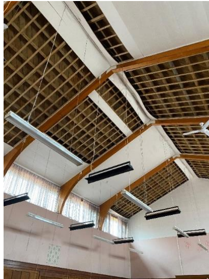
Figure 5. Roof structure over courtroom area
