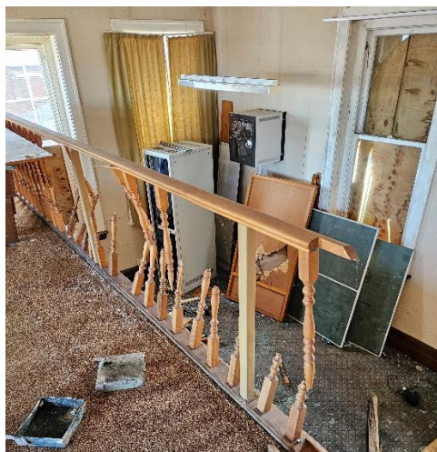
View of mezzanine
