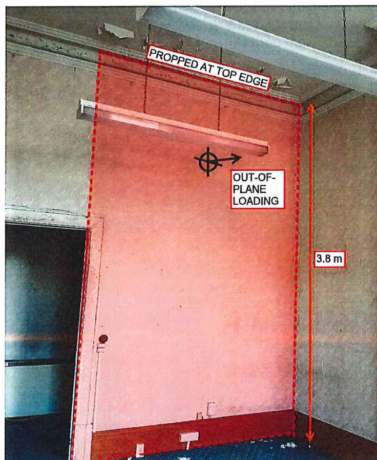
Figure 22. Out-of-Plane Loading on Internal URM Walls
