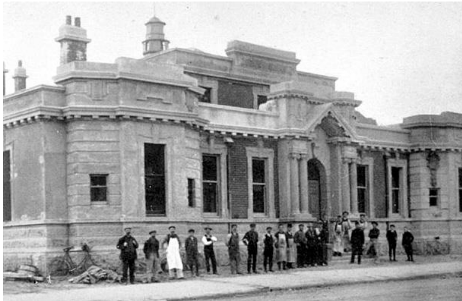
Original Building close to completion (note original parapet)
