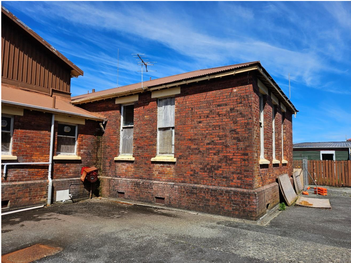
Rear brick construction
