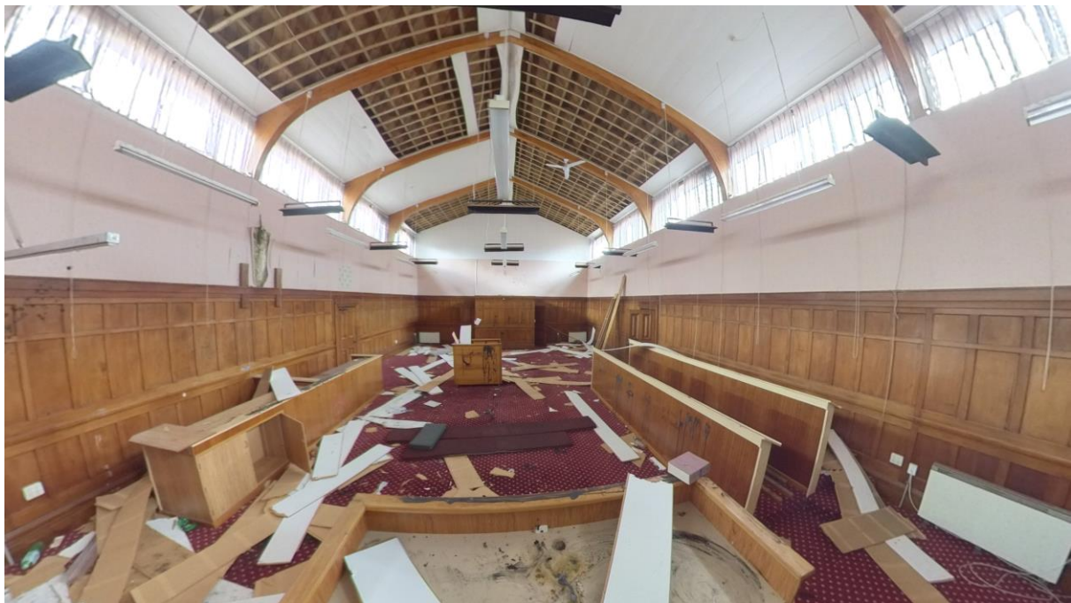
Figure 4 Courtroom timber interior
