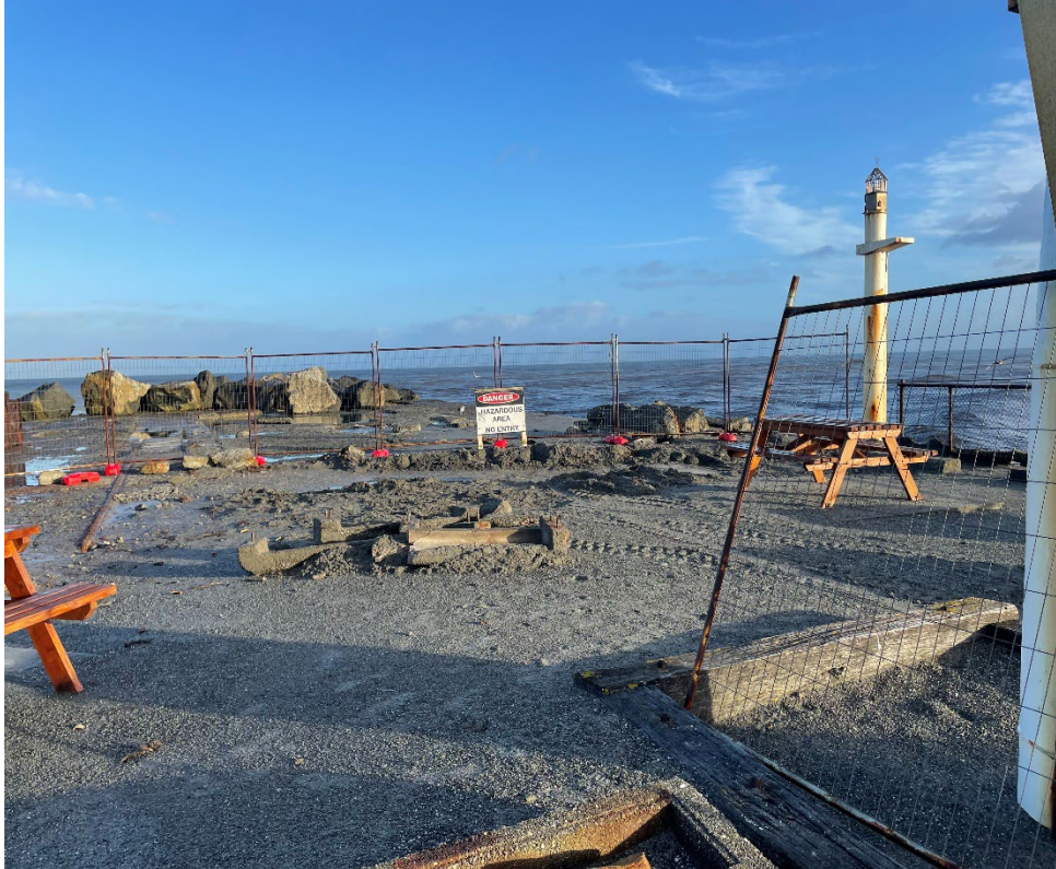
Figure 6 – Work in Progress
