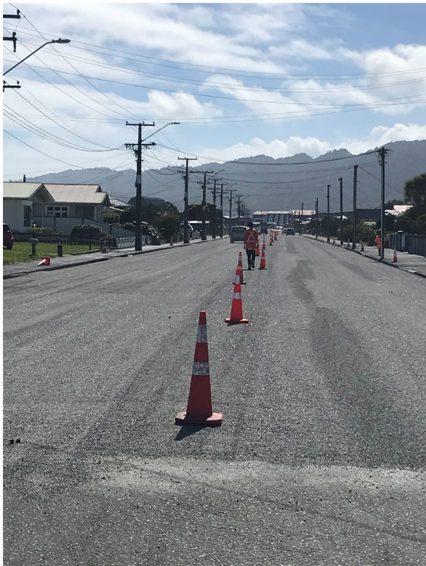
Figure 3: Re-sealing works completed on Preston Road
