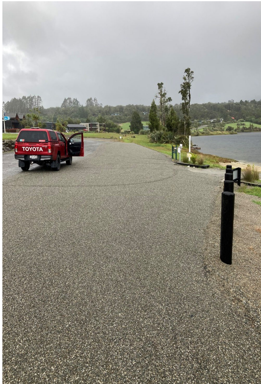
Figure 4: Iveagh Bay Boat Ramp Sealing
