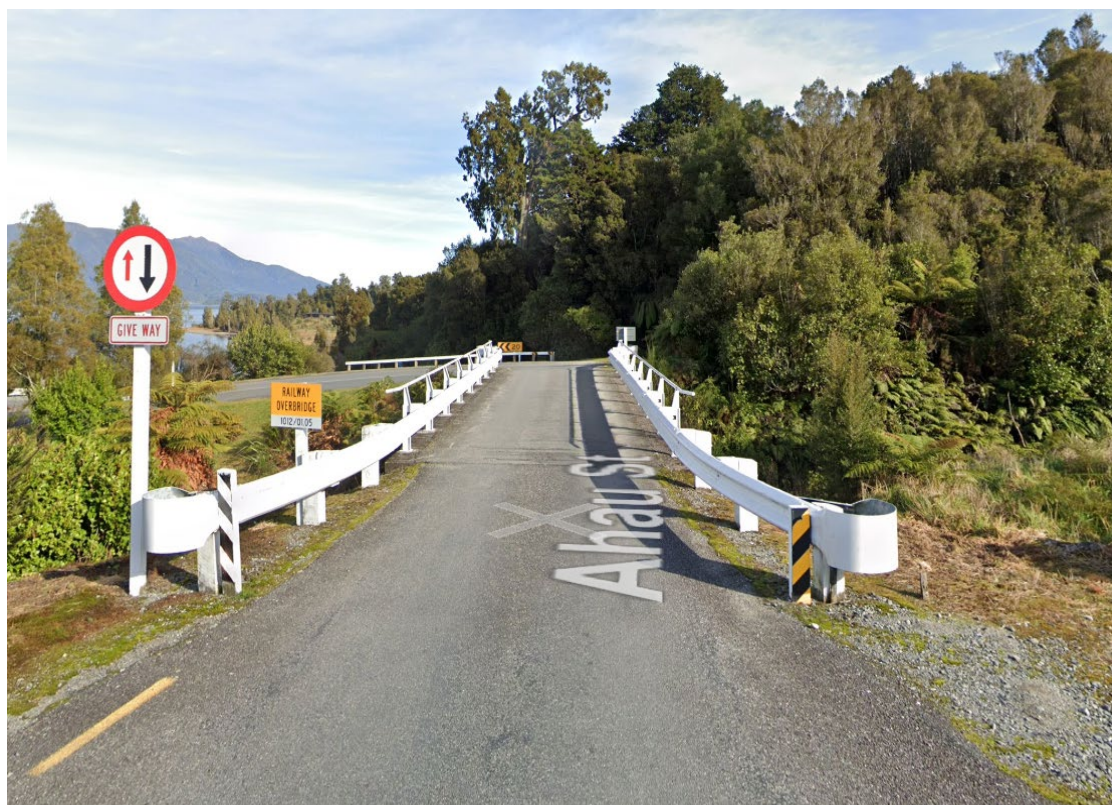
Figure 2: Speed Humps Programmed on Bridge
