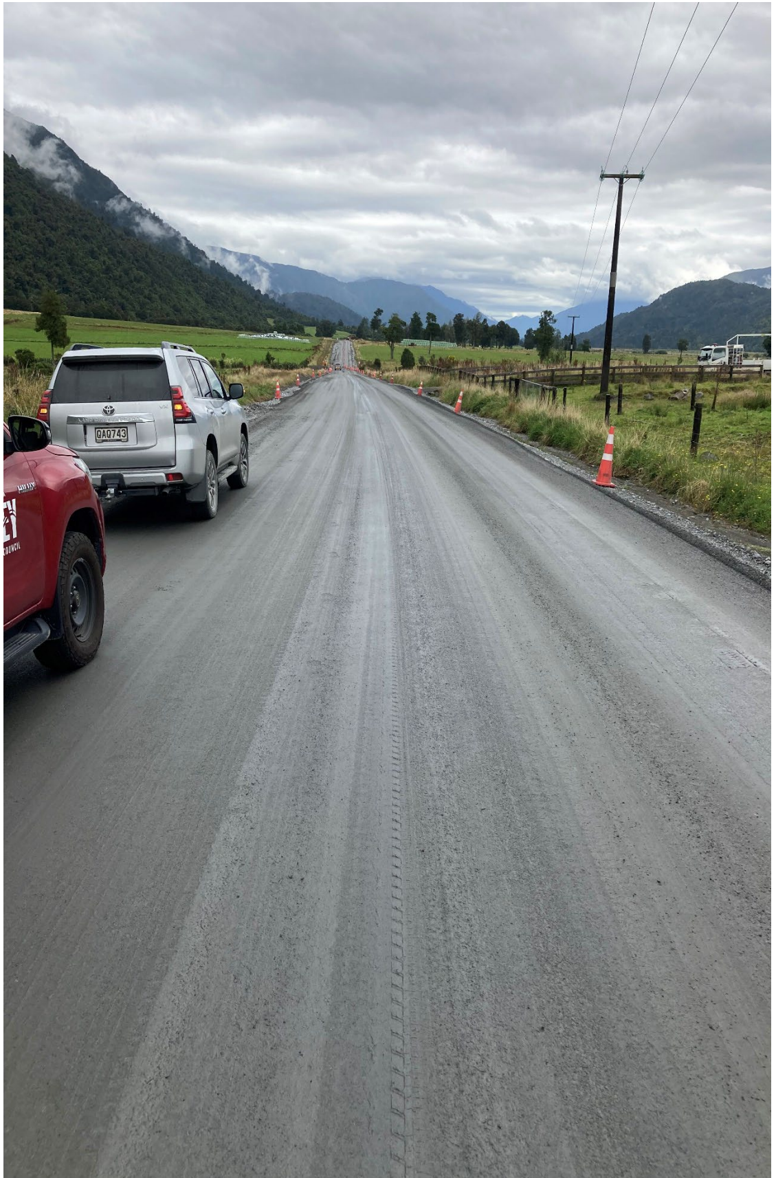
Figure 1: Pavement Rehab Works in progress on Lake Brunner Road
