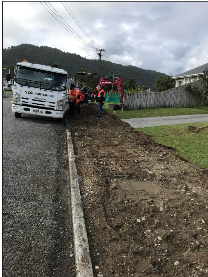
Figure 5: Mc Kane place Renewals underway
