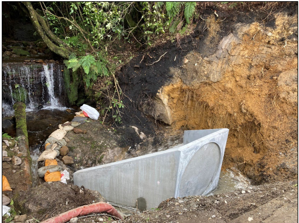
Figure 7: New headwall in place Taylorville slips site
