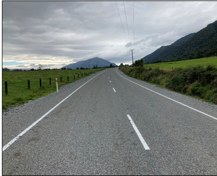
Figure 2: Lake Brunner Road Rehabilitation north-facing
