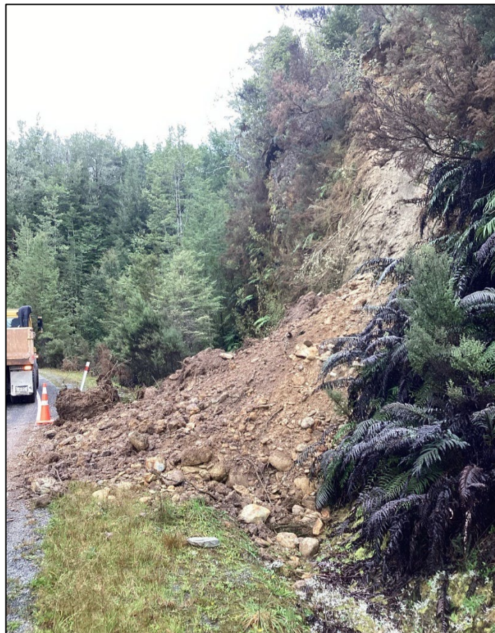
Figure 12: Minor slip Rutherglen Road
