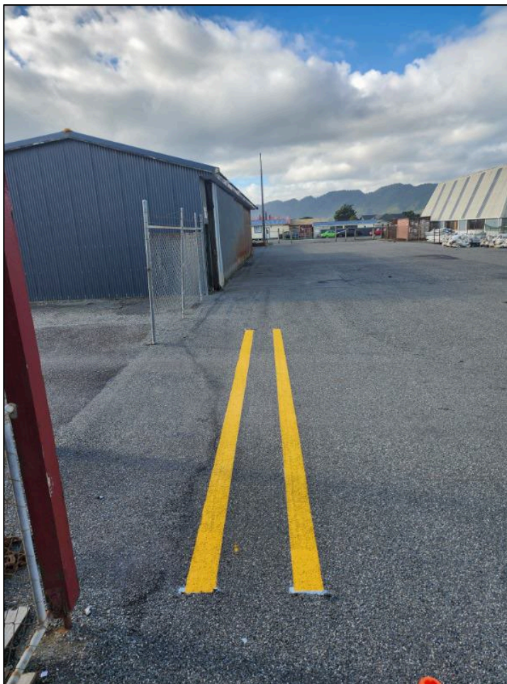
Figure 14: Taxi Way at airport remarked after sealing completed.
