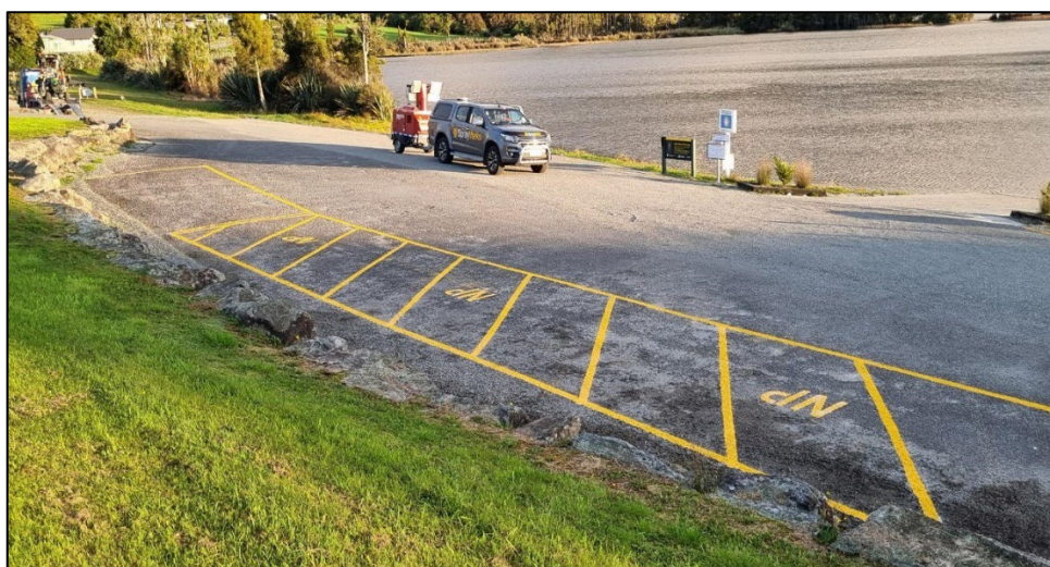
Figure 10: Iveagh Bay Boat Ramp Completed
