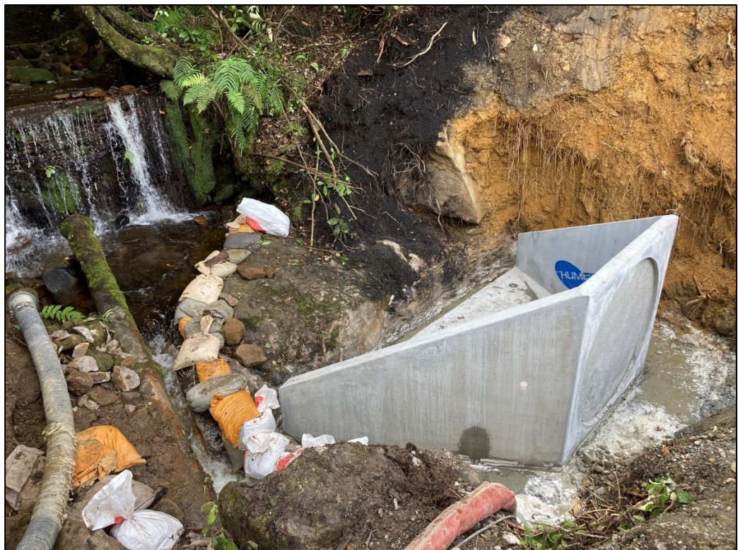
Figure 8: Controlling water while new culvert placed.
