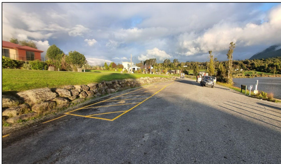
Figure 9: Iveagh Bay Boat ramp sealed and line marked
