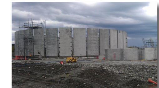
Construction of the Greymouth sewerage treatment plant, Preston Road
