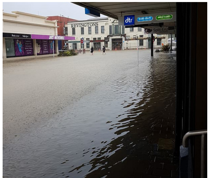
Flooding in Guinness Street, 11 January 2018 (ex Facebook) - the Greymouth CBD stormwater system is designed to cope with a 1-in-5 year on average storm
