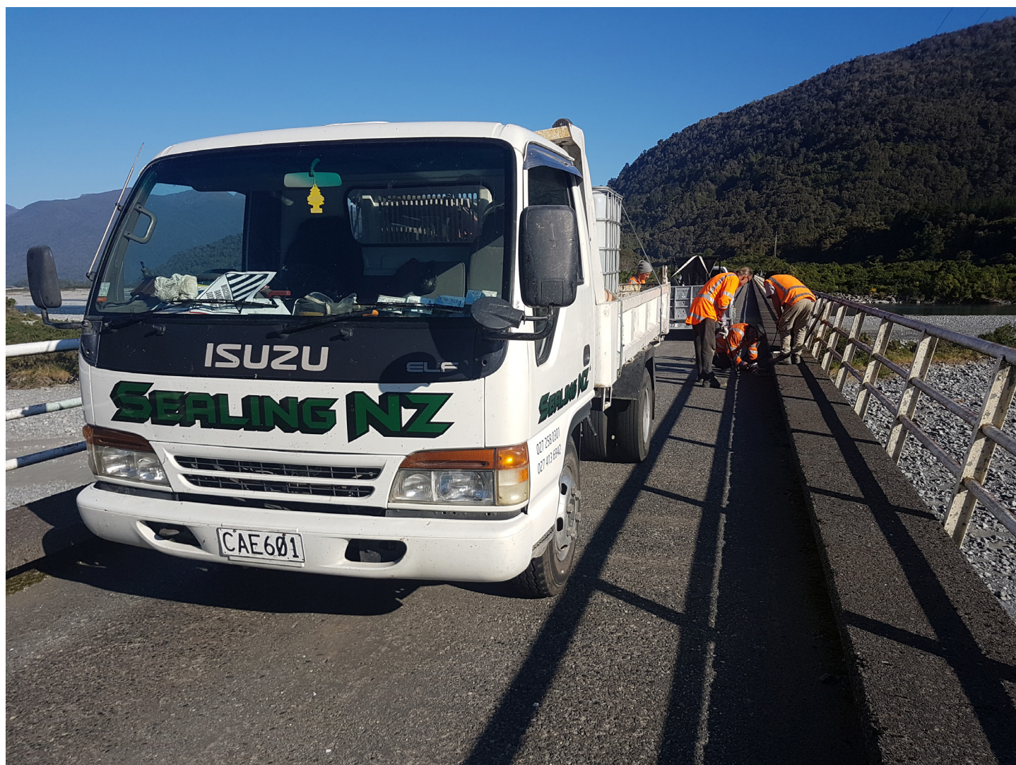
Contractors working on repairs to Stanley Gooseman Bridge
