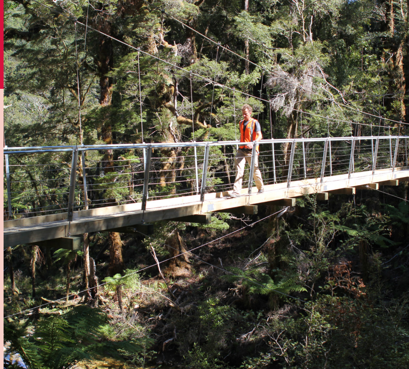
DOC Engineer Jono Calder inspects Watson Creek swing bridge
