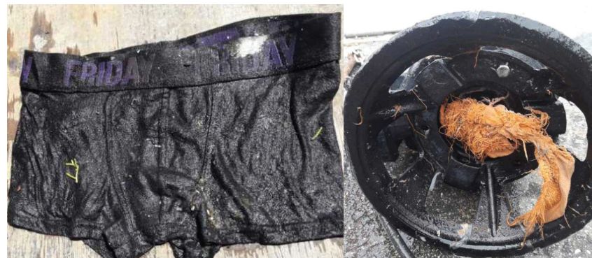
Some unwanted items recently found in our wastewater treatment plant
