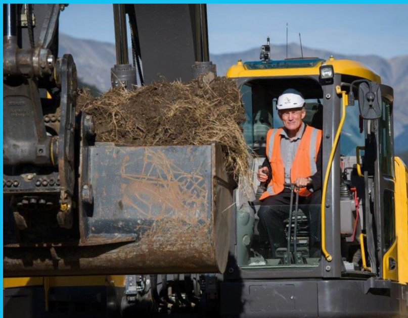
Mayor Tony Kokshoorn turning the first sod at Mingha Bluff
