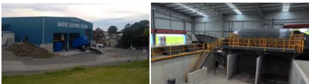
Figure 20: Marlborough Waste Sorting Centre 29
