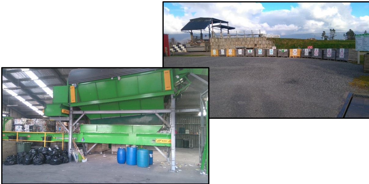
Figure 8: Westport Transfer Station - Drop-off area and MRF
