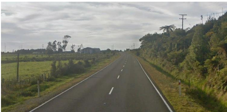
Figure 4: Existing Drainage Channel on SH6
